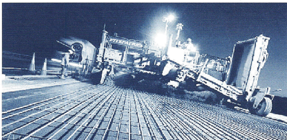
The working space needed is reduced by tipping the concrete onto a transverse conveyor that places it across the slab. On emptying a lorry, the conveyor lifts to allow passage of the next truck.
