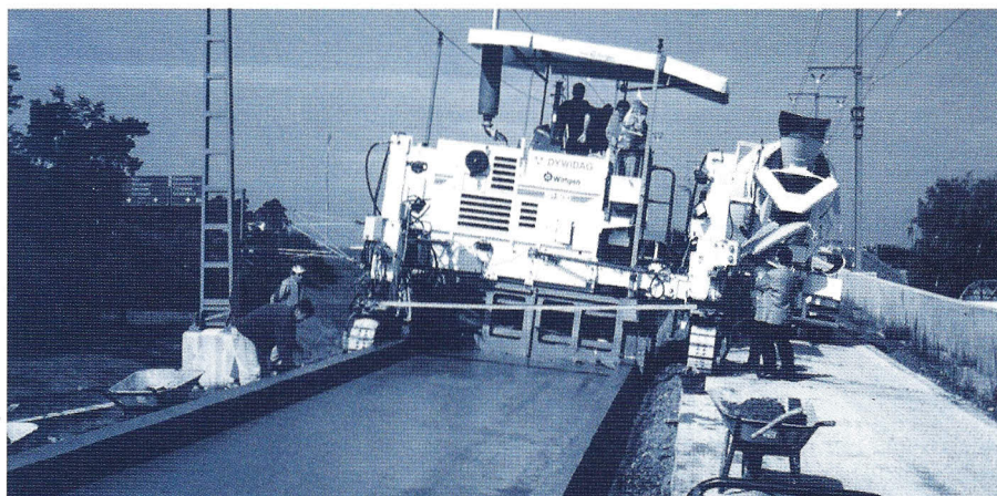
The Wirtgen paver at work on the Cologne-Frankfurt line, showing the 12% camber and side delivery of concrete supplies.
